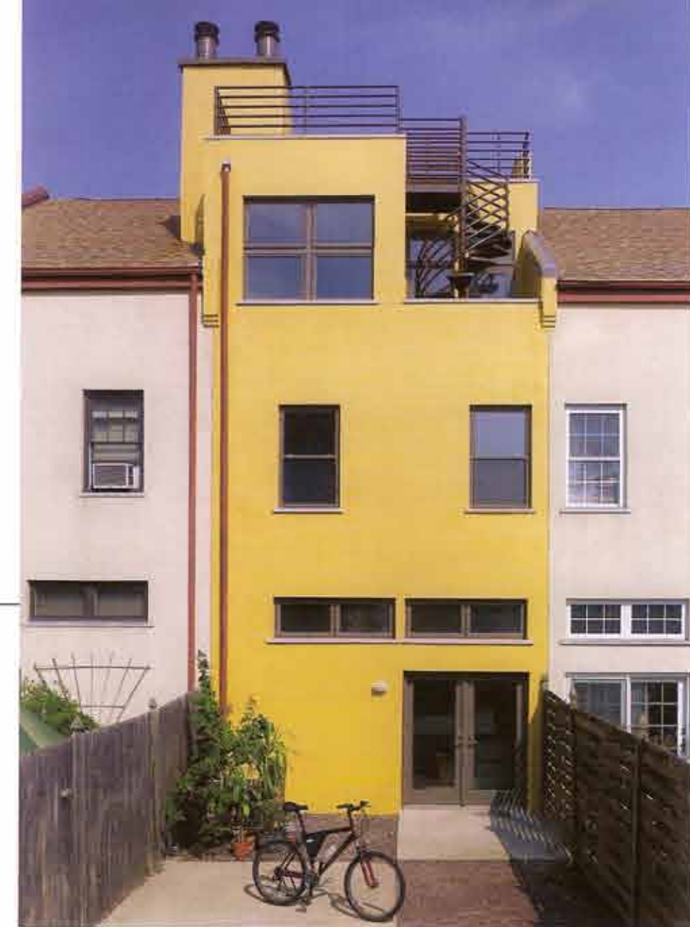
Above: The house, seen here from the parking court, was identical to its neighbors until the roof was removed to extend the structure upward. Photograph by Jeffrey Totaro
